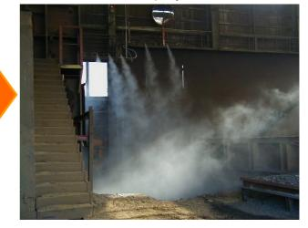
After the BIM spray nozzles were installed, the dust content was reduced by more than 90%.
